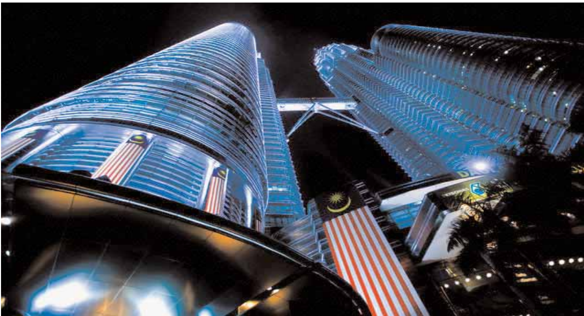
Kuala Lumpur - Le Petronas Towers
